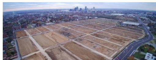
Future NGA West Headquarters site, 22 Sep 17
