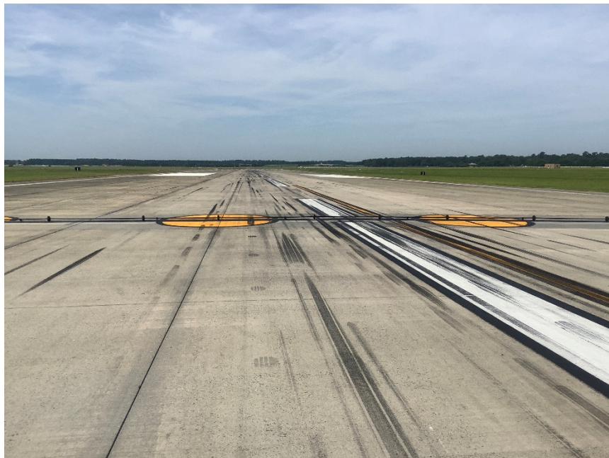
Figure 7: Runway 04L approach cable (Tab Z-10).
