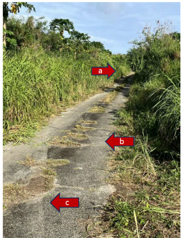
Figure 5: (a) Road narrowed by vegetation overgrowth, (b) and (c) MV tire marks departing road (view - opposite direction of travel) (Tab S-158)
