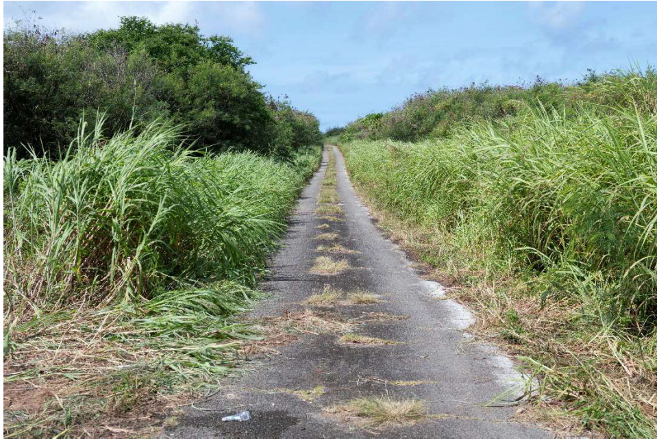
Figure 17 - Unnamed Road Where Mishap Occurred (Tab S-13)
